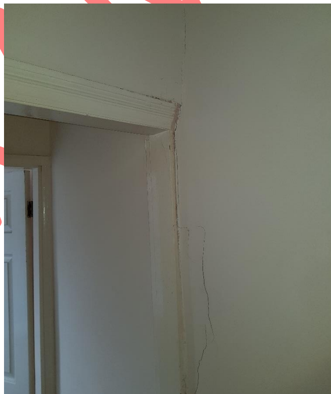
FIGURE 12 Cracking to the party wall at first-floor level.
