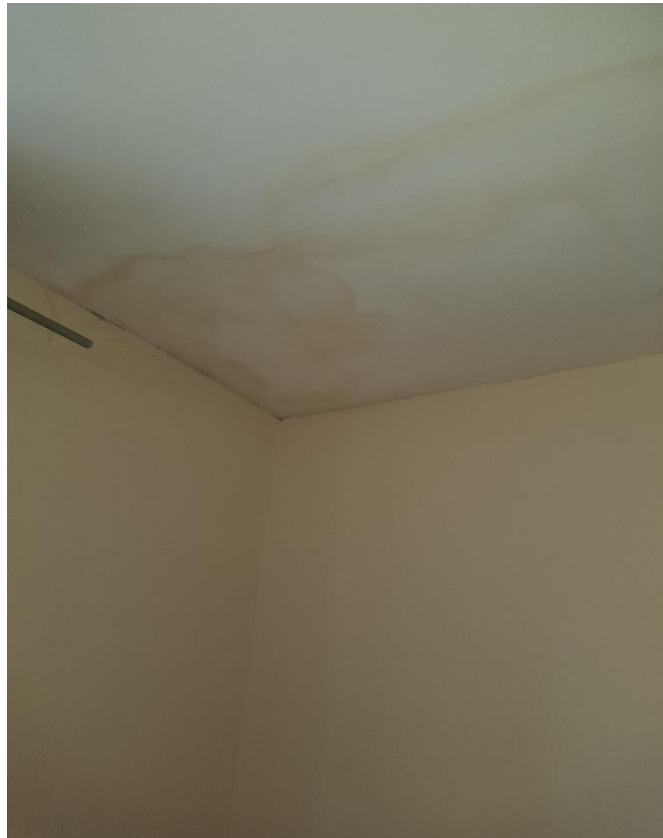
FIGURE 11 Discolouration of the front bedroom ceiling.
