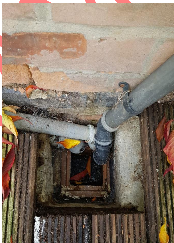
FIGURE 6 The blocked gully to the rear of the property
