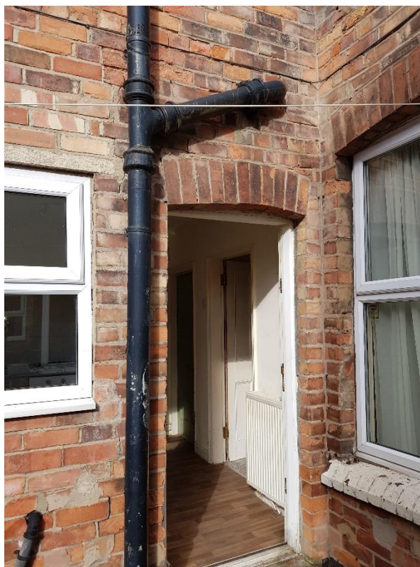
FIGURE 5 Lintel failure within the rear wing wall
