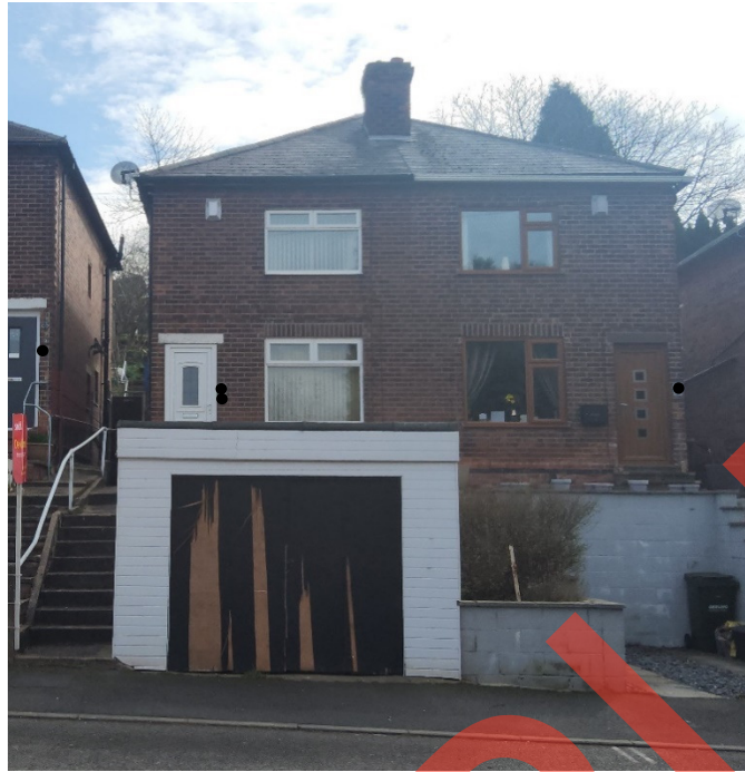
FIGURE 1 Photograph of the front elevation
